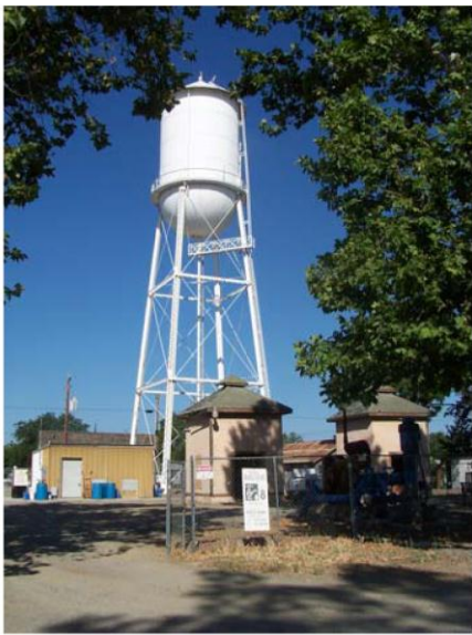
The City of Williams currently has one water storage tank located between Seventh Street and Sixth Street south of F Street.
