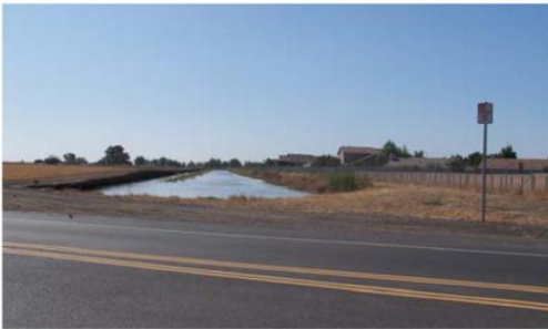
This detention basin meets engineering standards, serving only its drainage function.
