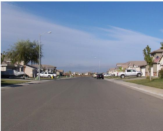
Most local streets in Williams have pavement widths of 40 feet or more. Future streets should be developed at the substantially narrower width of 28 feet.
