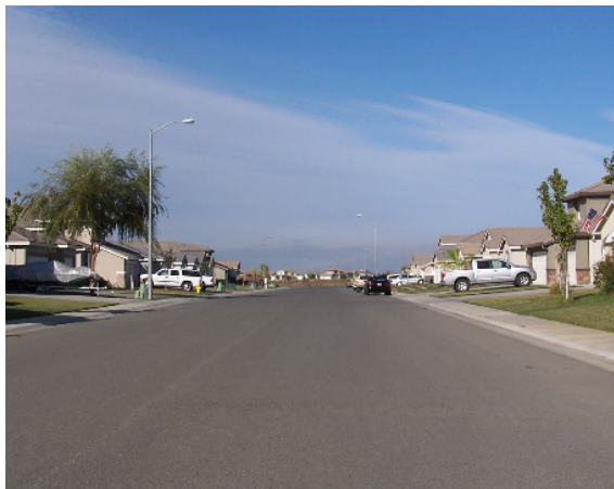
Most local streets in Williams have pavement widths of 40 feet or more. Future streets should be developed at the substantially narrower width of 28 feet.
